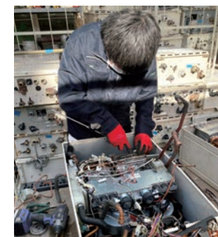
給湯器解体②
